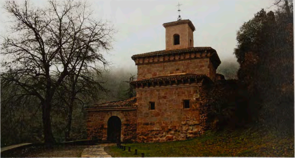
The tower of monastery of San Millán de Suso
