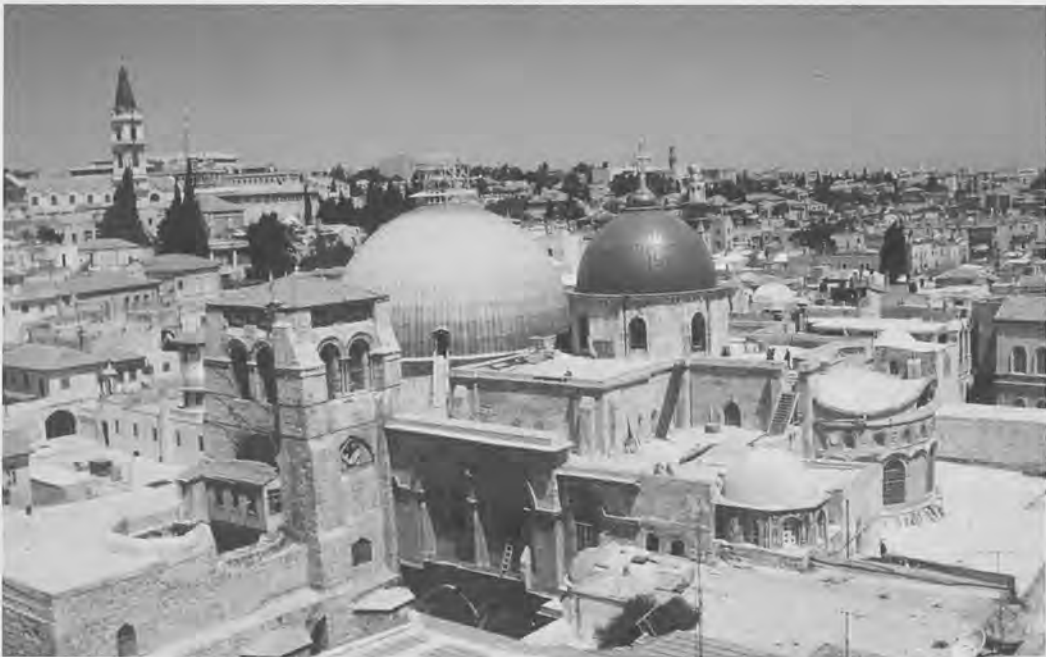
Fig. 1.- Church of the Holy Sepulchre, Jerusalem: view looking northwest (photo: J. Folda)
