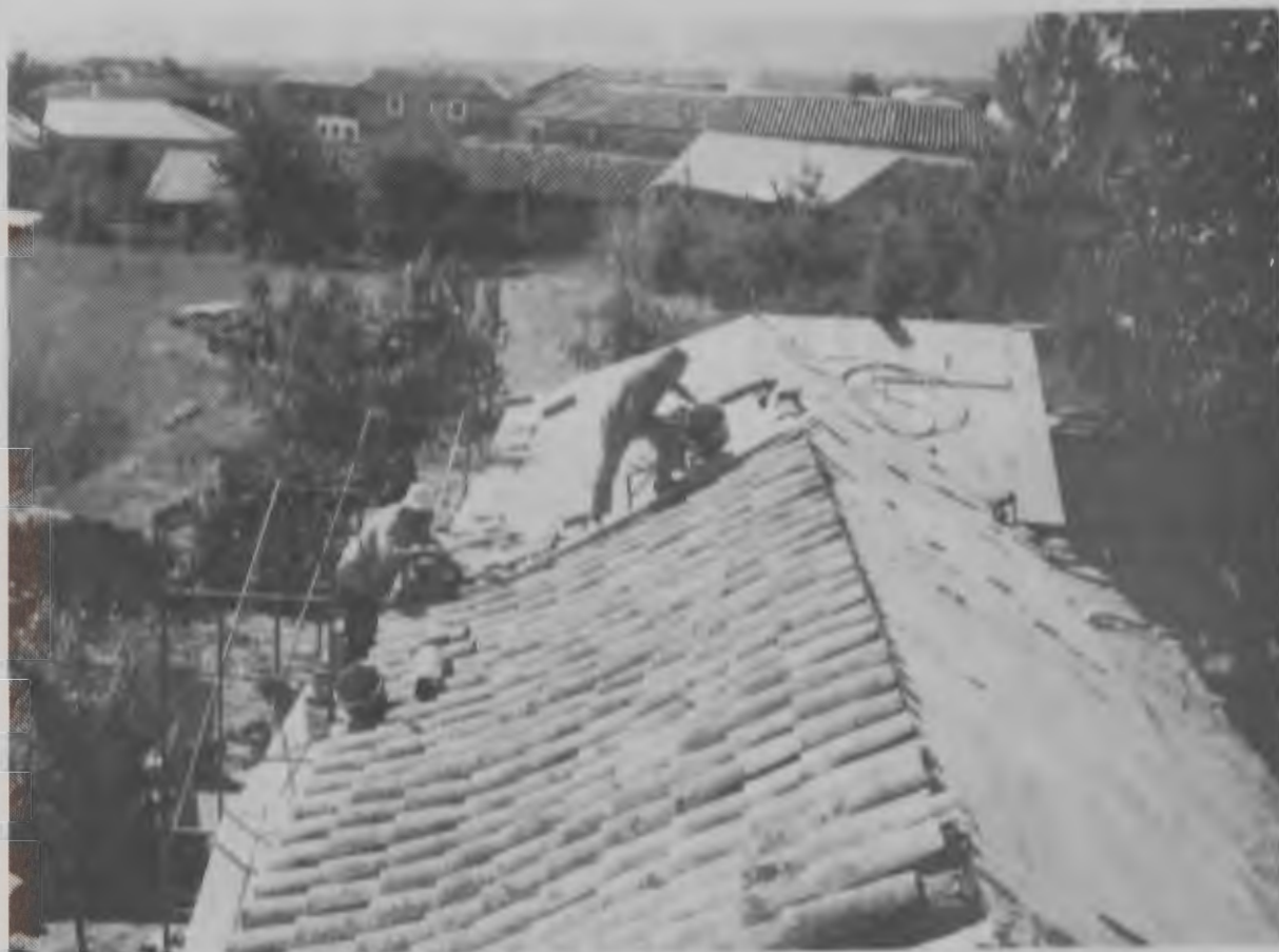
Halfway There: Tiles to the Left, Boards to the Right Photo: Barry Aston
