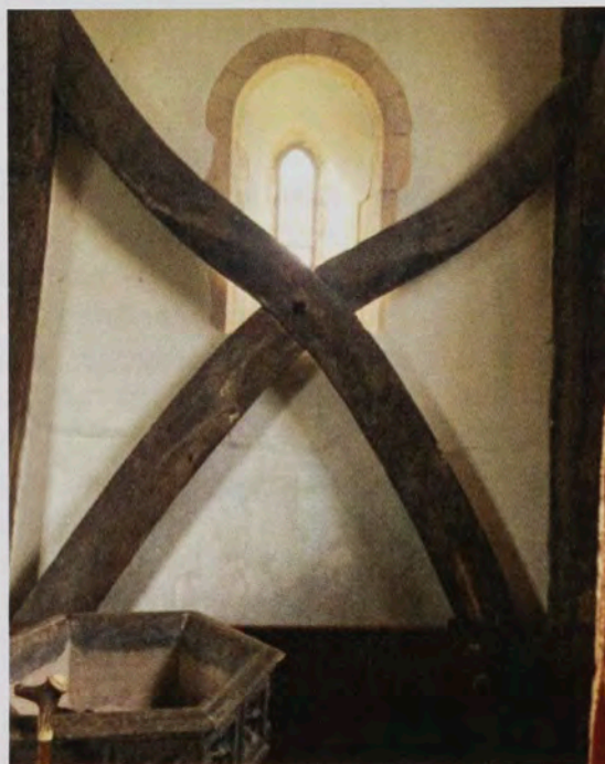
At St Mary's strange looking crossbeams support the bell turret and are believed to be unique in Kent.
