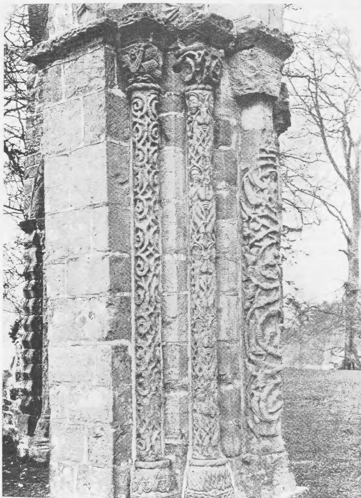
Fig. 2 The responds of the chancel arch: the Shobdon Arches (Photo: Royal Commission on Historic Monuments, England, Crown Copyright)
